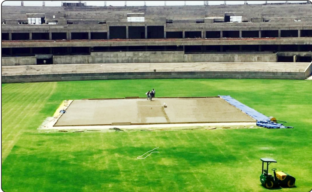
Structural work in progress at the New Stadium
