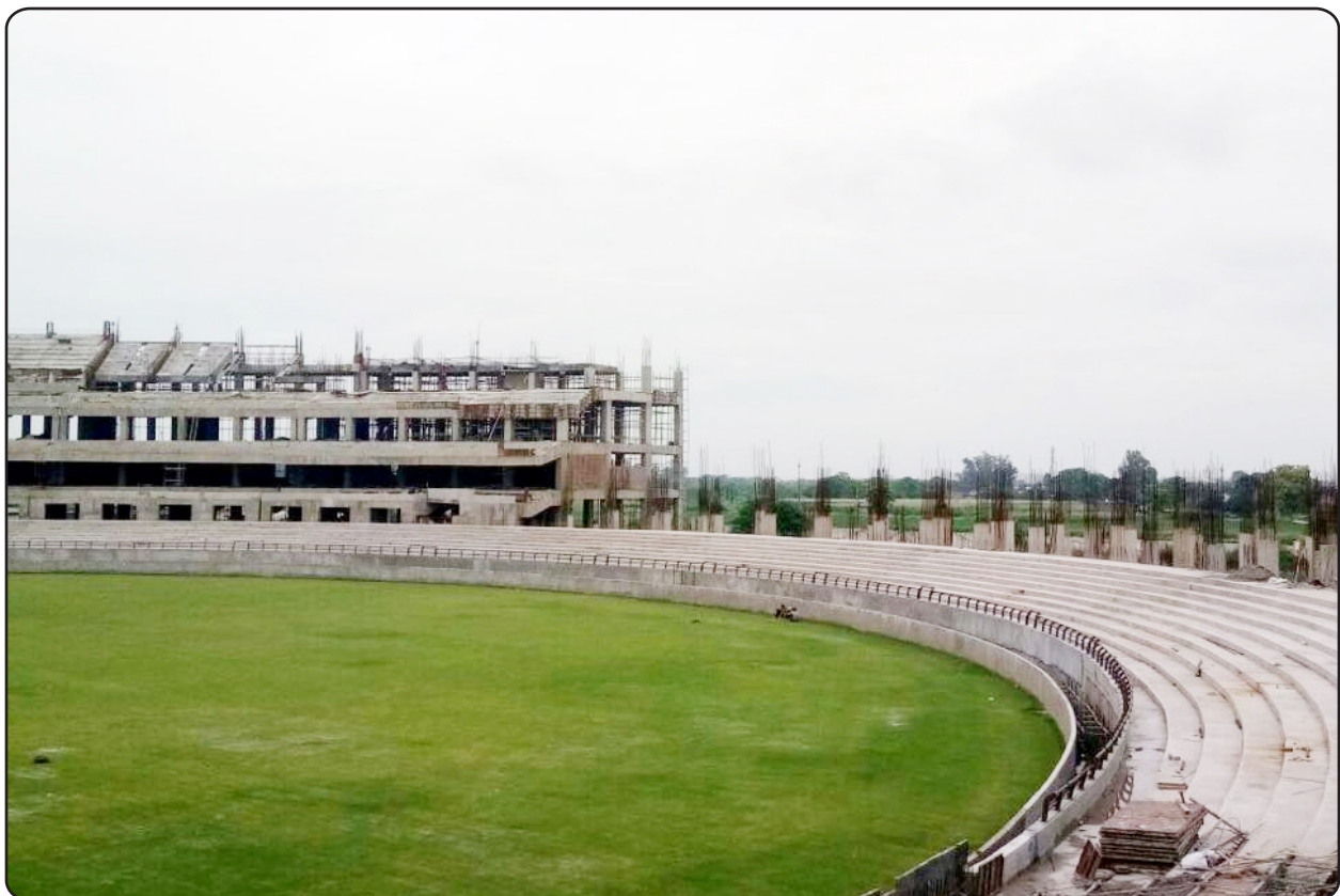
Structural work in progress at the New Stadium
